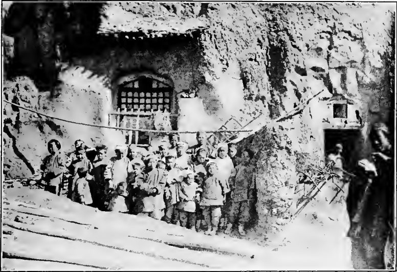
FIG. 43.—A vertical wall of loess in China with excavated dwellings. (G. F. Wright.)
